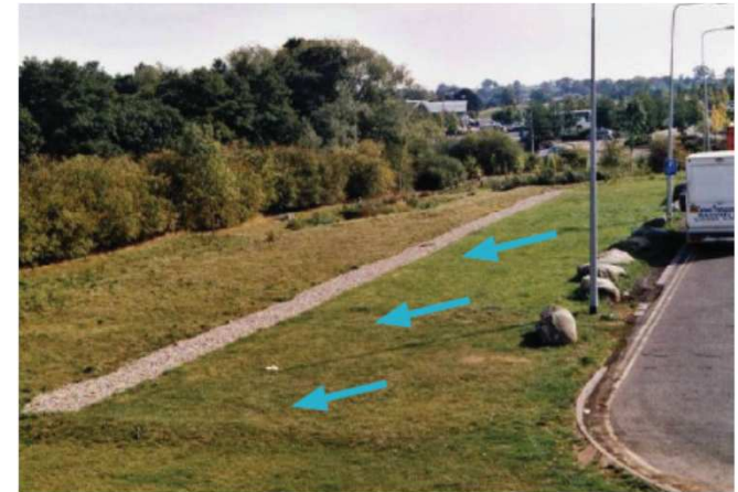
Filter strip leading to Filter Drain
